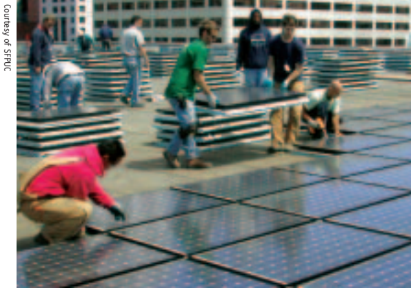
Workers install solar panels on the Moscone Center.
